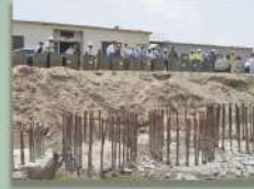
02 Progress review of Berth 15-17A project
