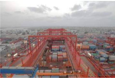
The Port itself consists of two wharves. The East Wharf has 17 multipurpose berths (Berth No. 1 to 17) and the West Wharf (Berth No. 18 to 30) has 13 berths. Each of the wharves has 2 dedicated container terminals with a design depth of 14 meters. The Karachi Port Trust has also three oil piers to handle liquid cargo.
